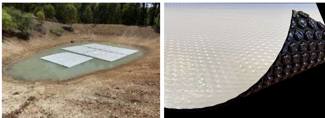
Figure 20: Daisy Dam cover installed as 5.24m by 5.24m square sections
