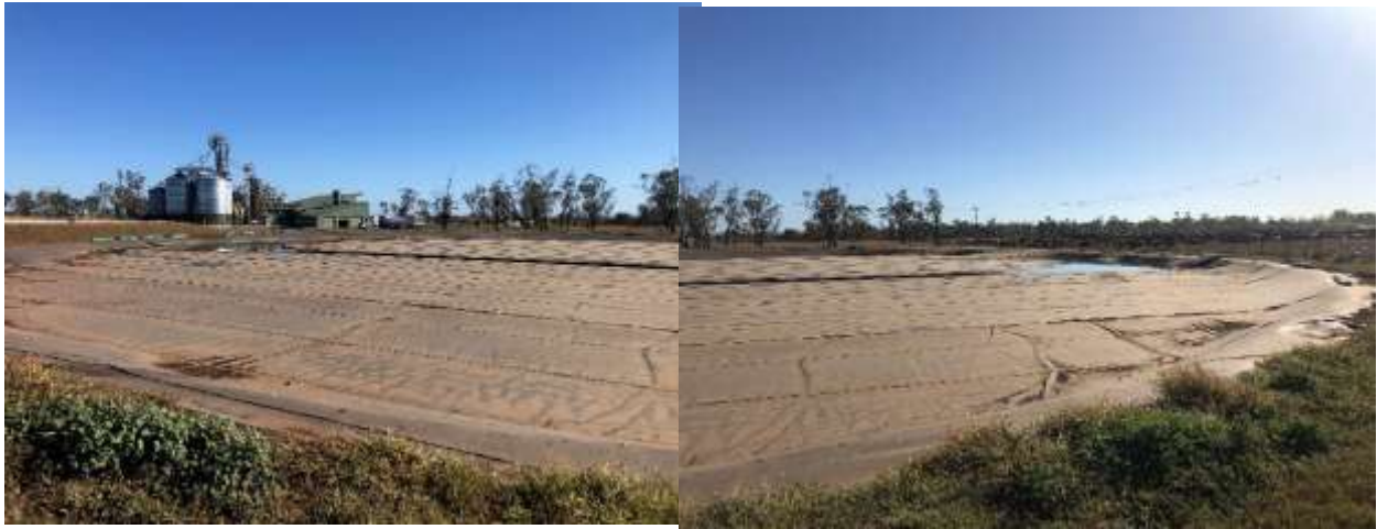
Figure 25: Aquacon Continuous floating cover installed at Wainui Feedlot (Photo: Matt Siebur)
