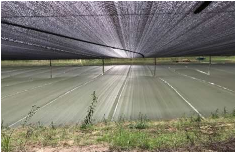
Figure 17: View from below a NetPro suspended shade cloth cover at Stanthorpe used to reduce evaporation and increase security of supply to irrigated apple orchards.
