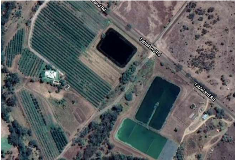
Figure 29: Aerial photo of Gayndah sewerage treatment works
