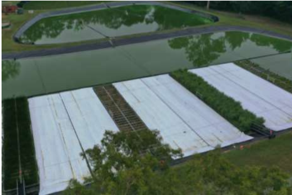
Figure 30: Daisy Dam Cover over a treated effluent pond in Kenilworth Queensland (photo: Clarity Aquatic)
