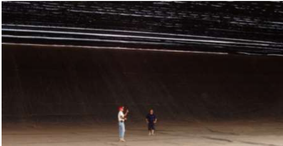
Figure 8: A double-layer black woven polyethylene cover over a lined reservoir in Spain
