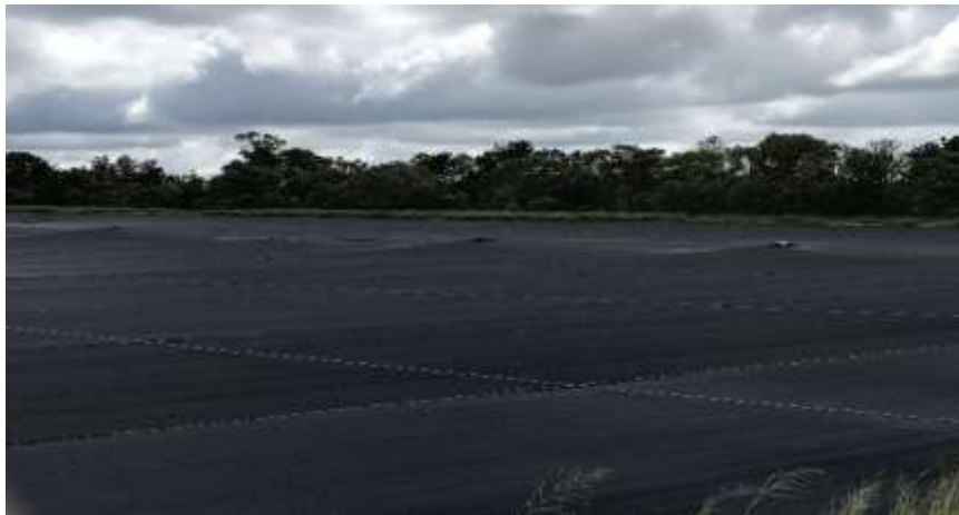
Figure 28: NetPro Shade cloth canopy over an irrigation water storage (photo: Erik Schmidt)
