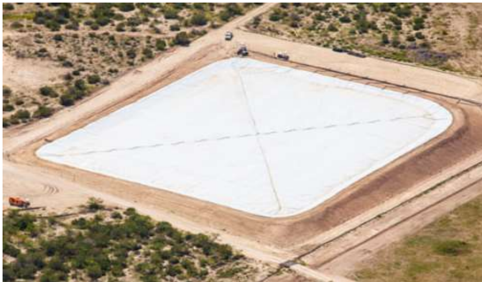
Figure 18: Example of a Layfield continuous floating cover
