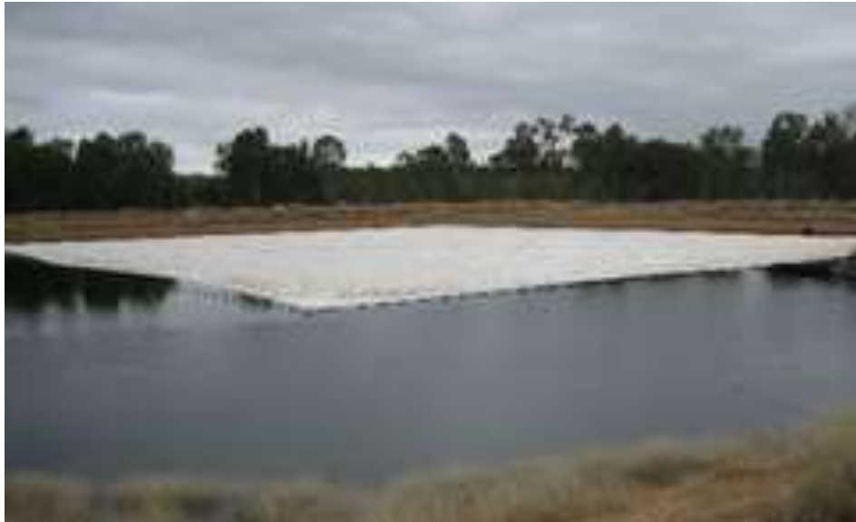
Figure 27: Partial coverage of the storage at Redbank Plantation with an EvapCap continuous floating cover.
